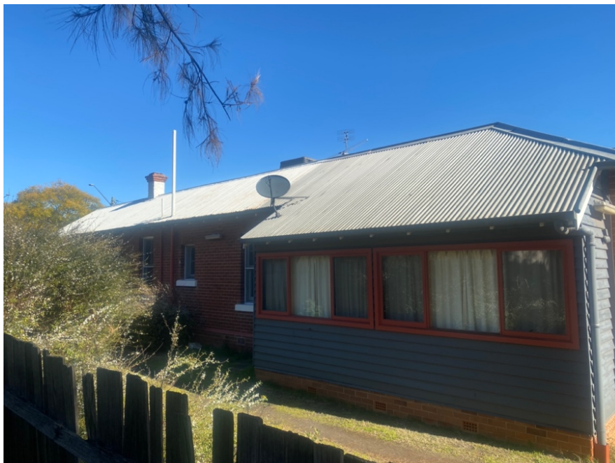
Photograph of the northern side of the building showing the junction between the original cottage and the 1980 extension. There is a noticeable difference in the roof colour and this part of the extension is clad in clapboard. (Ray Christison 10.8.2022)
